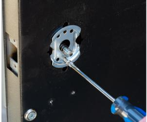
If the door was previously prepared with a 2  $\frac{1}{8}$ " face bore, use the retrofit mounting plate and screw to secure the bottom post of the front lock housing.
