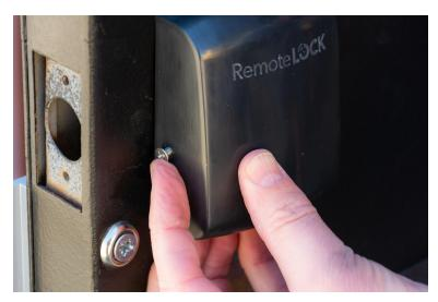
Secure with a small screw on each side of the cover.
