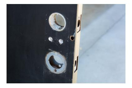
Using the drilling template, prep your door to fit the exit bar lock mounting hole requirements. Door pictured here was previously fitted with a lever and deadbolt, so a cover plate will be utilized to cover old cross bore holes.
